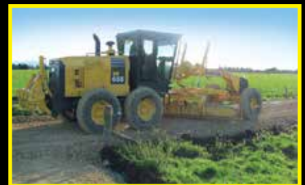
Road Construction and Lime Capping
