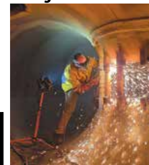
Above: cutting the stay bolts inside the old turbine
